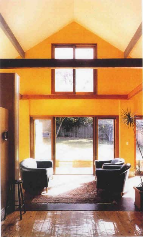
Left: Beams and ceiling of the back extensions are now in place for the proposed loft bedroom. This will be completed during the second or even third stage of the renovation, according to family needs. The important point is that nothing in place now will need to be demolished or altered to allow for newer work. Above: The previous view from exactly the same place!
